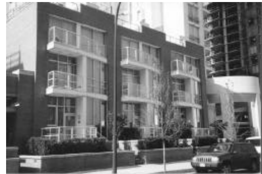
Three-Storey Townhouses: Marinaside Crescent
